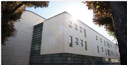
The Veterinary University Hospital at Maison-Alfort
